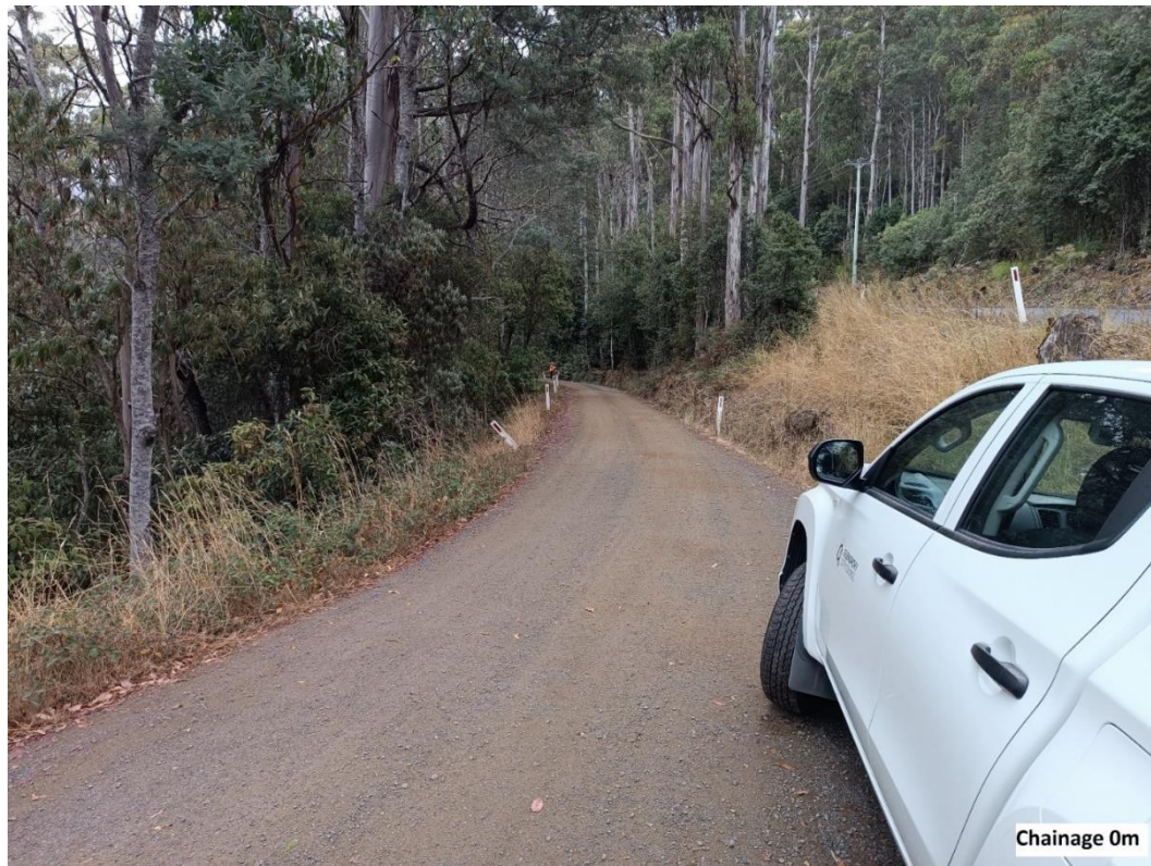
Ch.0 - Sight Distance: 80m. Road Width: 7.2m Ch.100 - Sight Distance: 70m. Road Width: 3.2m
