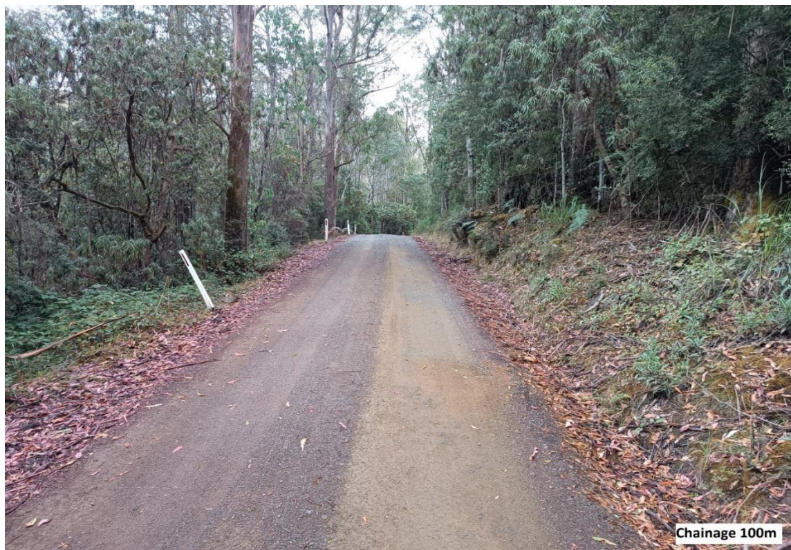
Ch.0 - Sight Distance: 80m. Road Width: 7.2m Ch.100 - Sight Distance: 70m. Road Width: 3.2m
