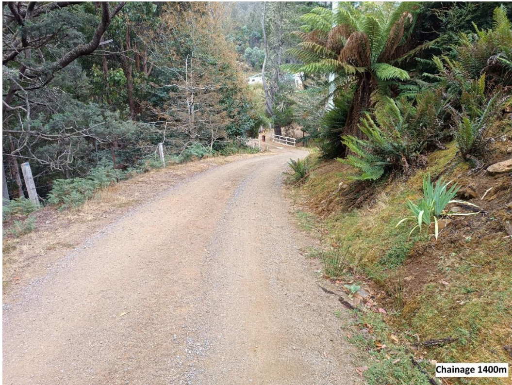
Ch.1400 – Sight Distance: 60m. Road Width: 3.4m Widened section at Ch.1460 (Between bridge and parking area)
