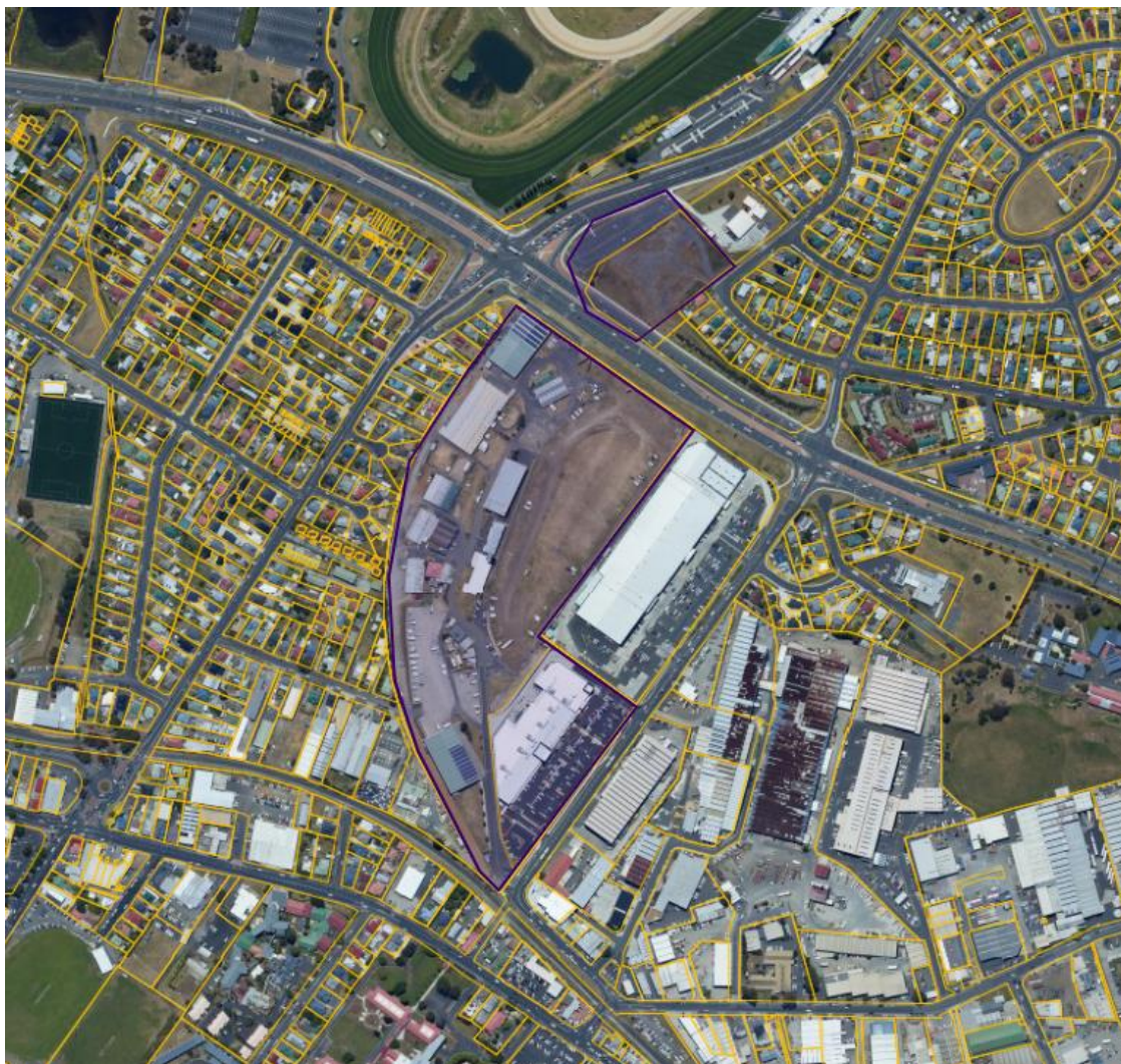
Figure 3: An aerial view of the site and surrounds with the application site highlighted in purple (Note, several of the existing buildings at the site shown in this aerial image, have been demolished)
