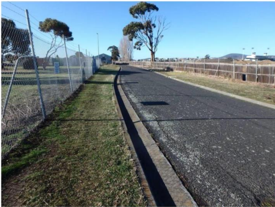
Plate 9: View east along Loyds Lane in the northern portion of the study area, obscuring the natural soil deposits
