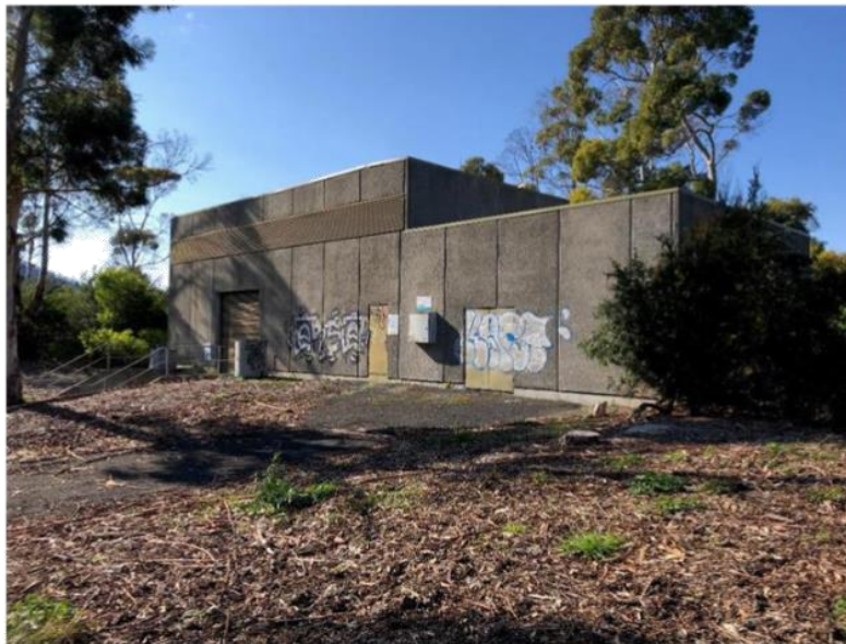
Figure 7: TasWater's Elwick Water Pumping Station at 559 Brooker Highway (HOBWP15)
