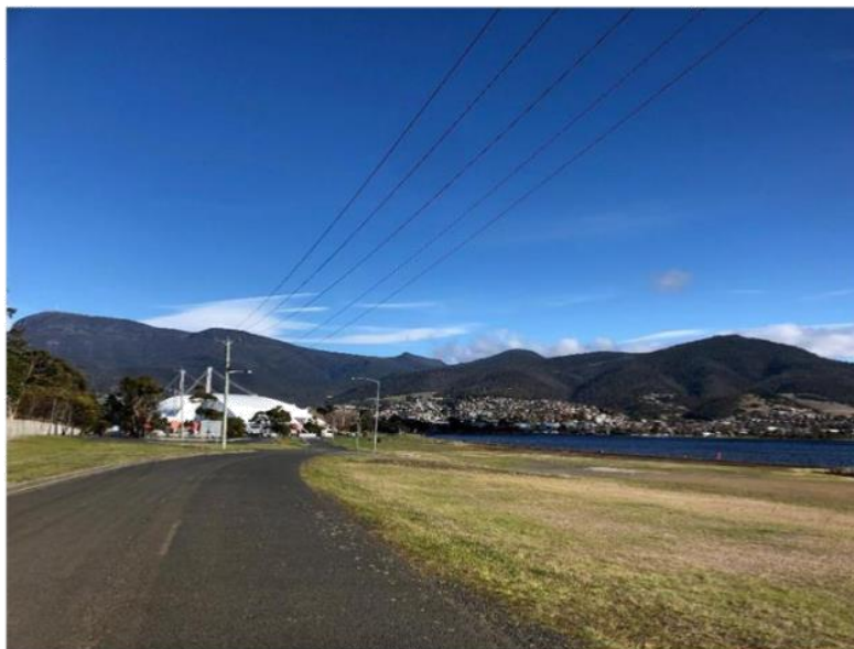
Figure 8: Overhead powerlines running from north to south, terminating at the DEC building
