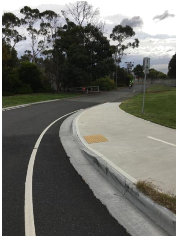
Photograph 3: Showing the slip lane taken towards the Wilkinsons Point site
