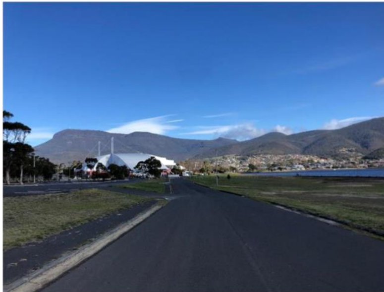
Figure 9: Existing road through #601, with overhead street lighting
