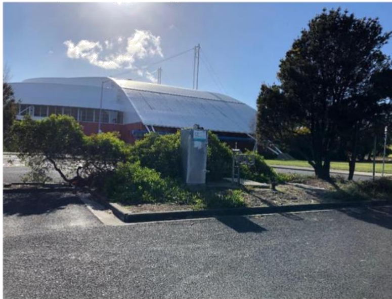
Figure 6: TasWater's DEC Carpark Sewage Pumping Station (POWSP03)
