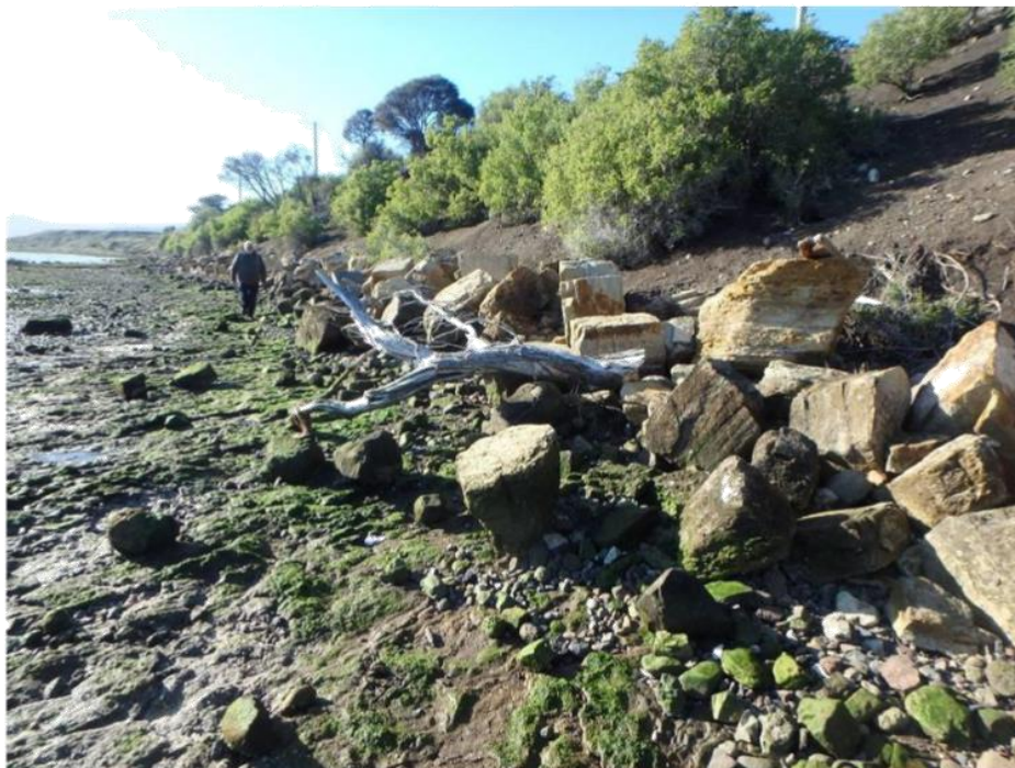
Plate 5: View north-east along the rock platforms and tidal mud flats in the intertidal zone at Wilkinsons Point, with rock bubble fortifying the embankment
