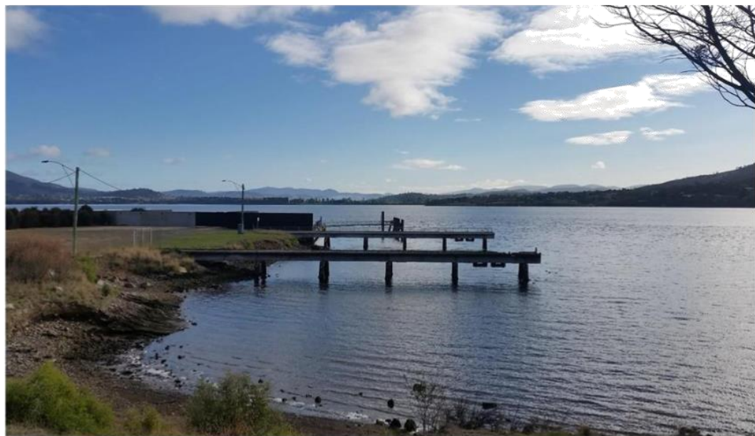
Figure 23: Existing jetty piers at Wilkinsons Point with access to ferry services.
