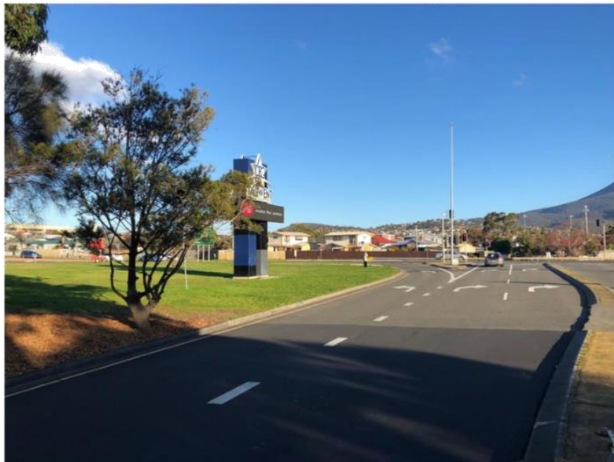
Photograph 5: Intersection of Wilkinsons Point Access Road and the Brooker Highway
