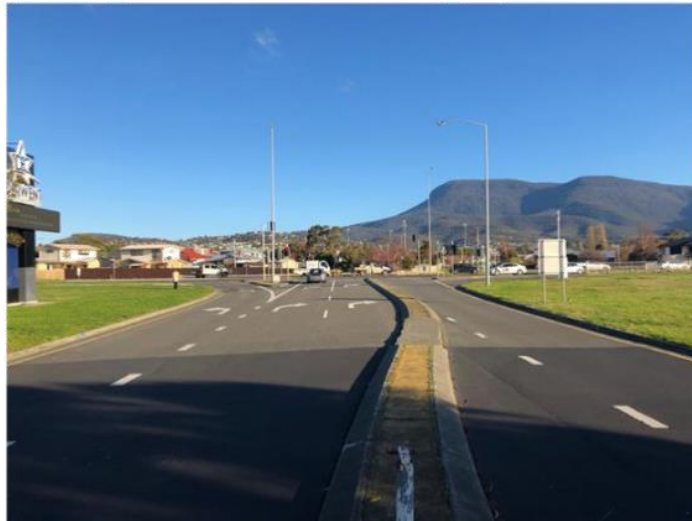
Photograph 1: Showing the Wilkinsons Point intersection with the Brooker Highway
